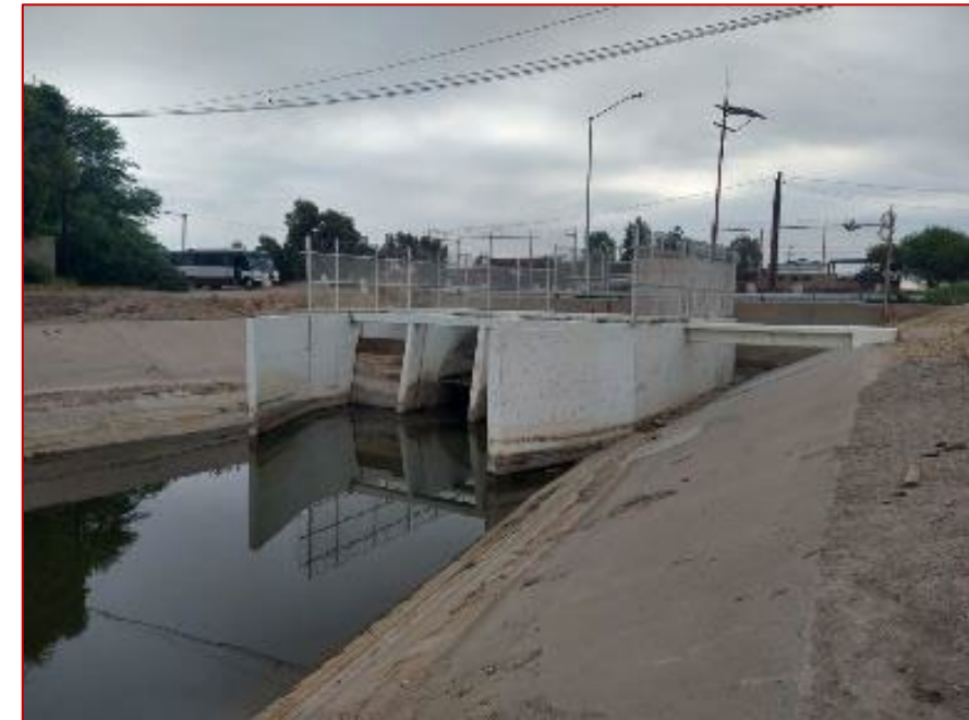
Weir modernization project in Mexicali irrigation district
