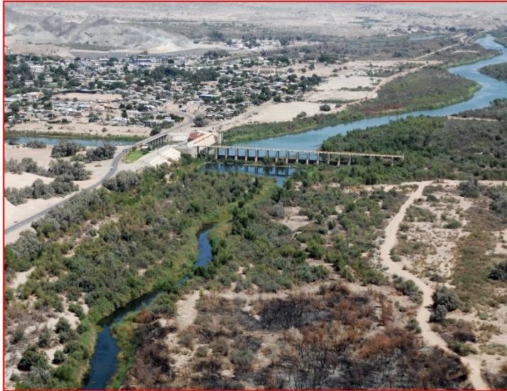
Colorado River at Morelos Dam at US-Mexico border
