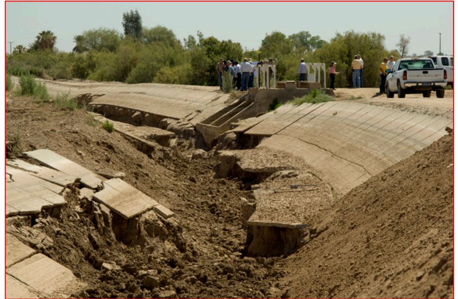
Earthquake-damaged canal in Mexico
