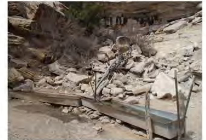
65 Water-Safe Spring, an unregulated water source on the Navajo Nation, water is collected and funneled to watering troughs downhill of a spring. Source: Joseph H. Hoover.
