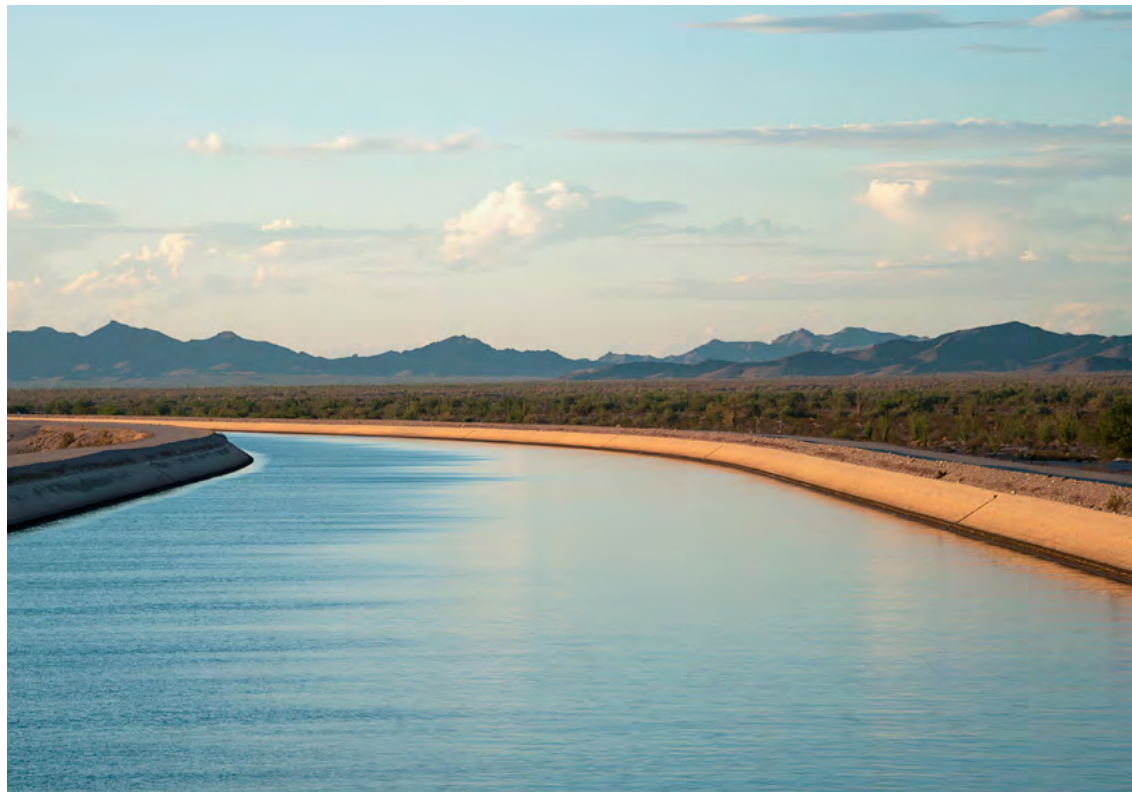
CENTRAL ARIZONA CANAL
