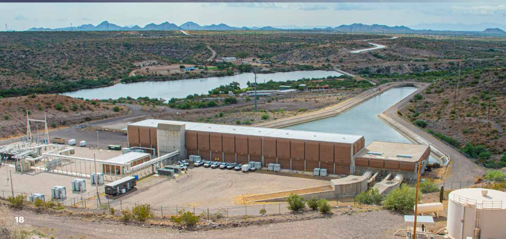
Waddell Pump/Generating Plant
